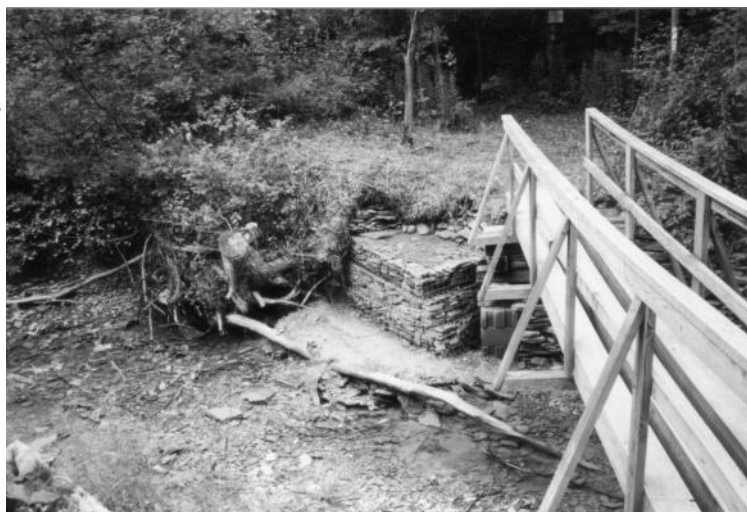
Bridge in Shindagin Hollow State Forest after gabions (rock-filled wire baskets) were installed on August 20.
