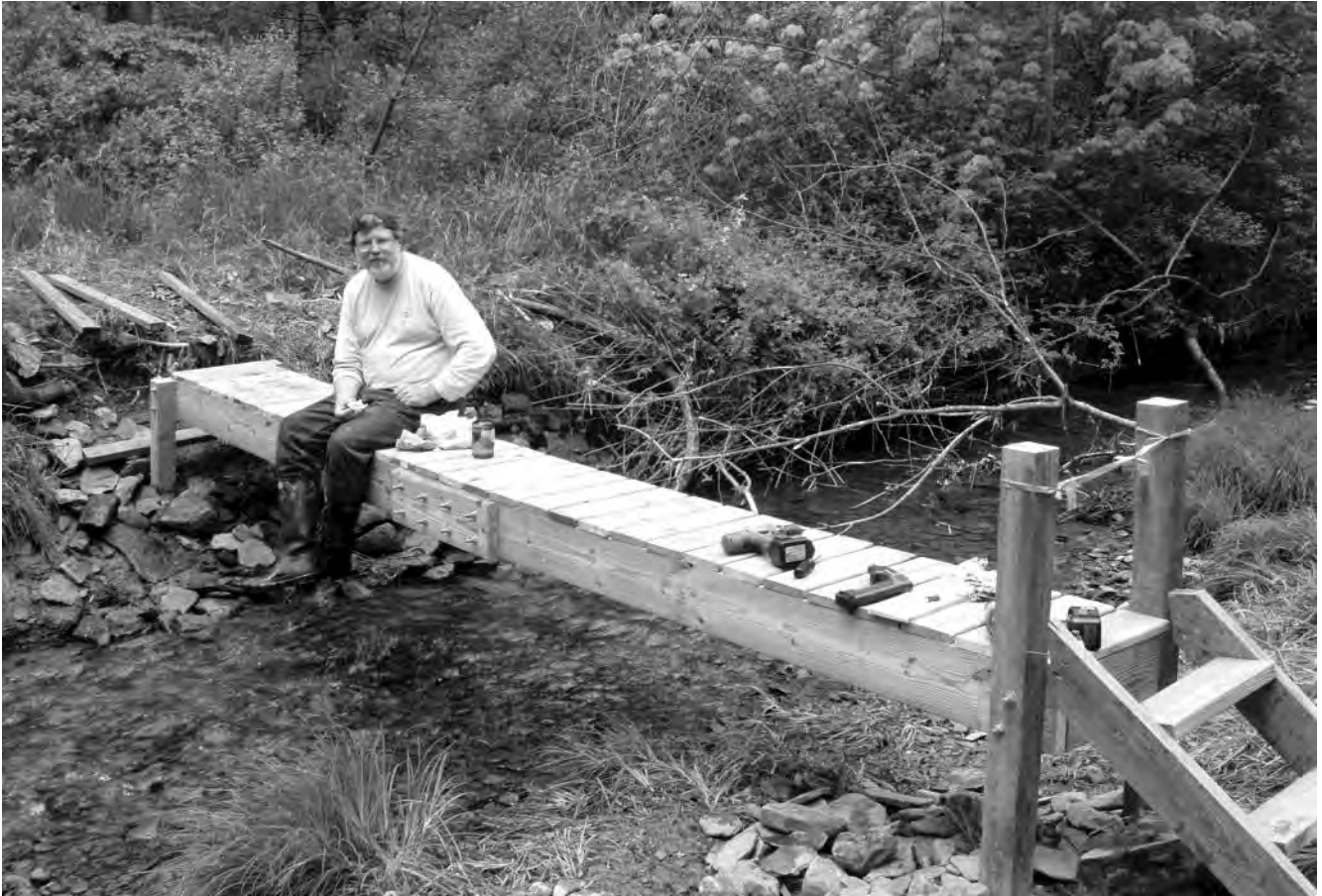
Bridge over Logan Creek. This photo shows the "sandwich" compression bridge joint and the anchor supports. That's Greg Lawrence seated on the bridge.
