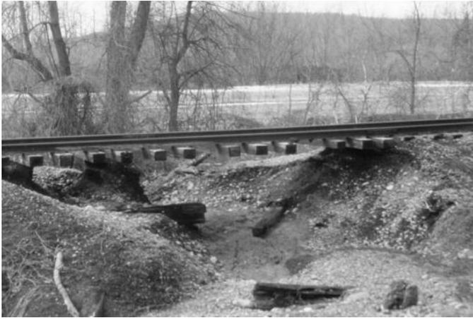
*Built-up railbed completely washed out beneath tracks, south of Brisben. Swollen streams crashing down eastside hills burst across the road and tracks last June, undermining tracks in some places, burying them in dirt and rocks in others.*
