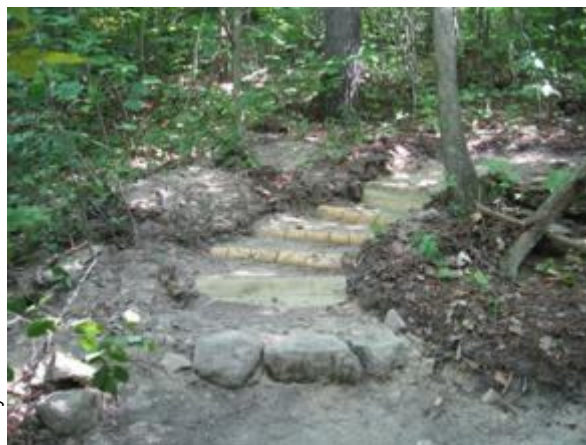
New steps on the steep trail up Mt. Washington near Hammondsport. When the crew ran out of pressure treated wood, they used black locust and stones for steps.
