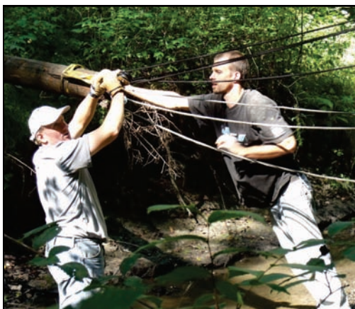
Above: As the pole is inched across the creek, Mike Schlicht and Jason Benedict attach extra pulleys and lines to keep the pole's nose up. Photo by Leona Jensen
