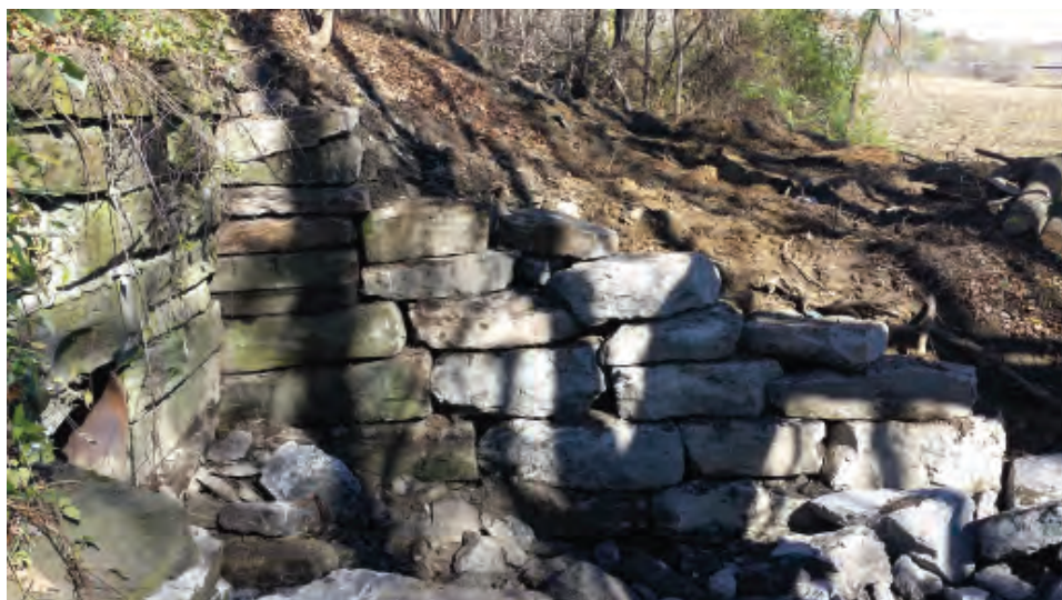
The right wing rebuilt and extended approximately 10 feet.
