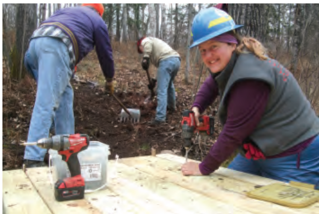
Here Jo is decking a long bridge the Wisconsin Rovers Crew built along the North Country Trail.
