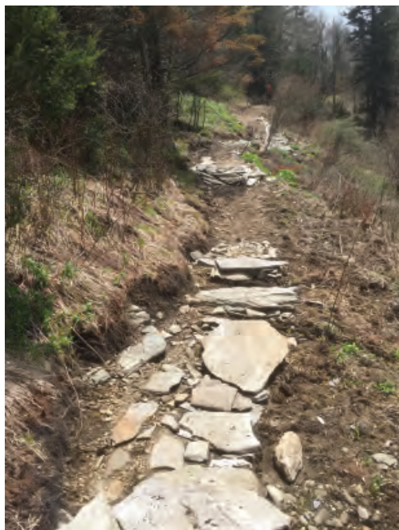
New trail intermittently “paved” with slabs and rubble. Plenty of rock material available there!
