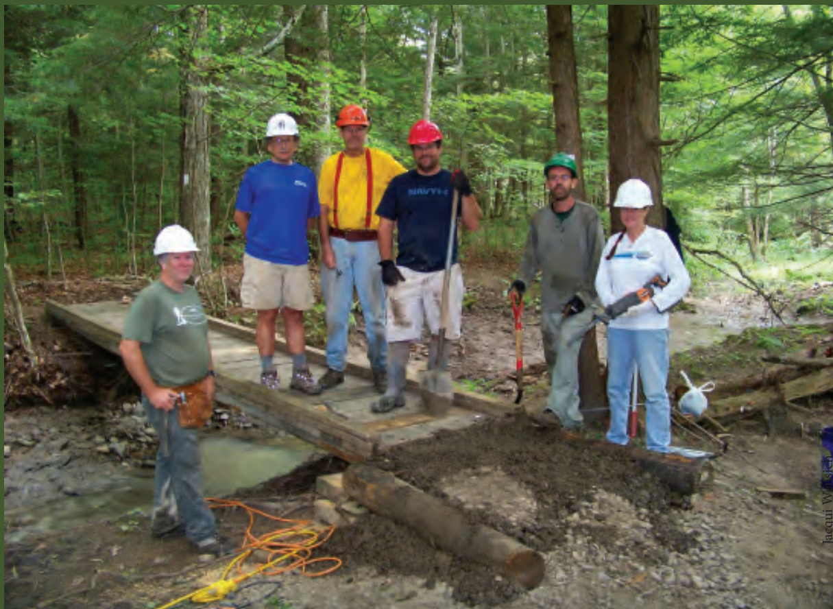
Birdseye Hollow crew at repaired bridge, now clear span across the waterway with no center support to snag debris. Notice steel cables tied around trees at each end, and the ramps made of stream gravel. Left to right, Mike Ogden, Dave Newman, Bob Emerson, Kenny Fellers, Steve Catherman, and Linda Ratsep.
