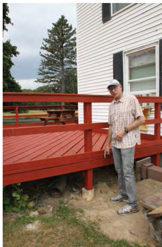
AFTER: Mike cut off the old rotting deck, redid the supports under the new edge of the front deck, and stained the whole thing.
