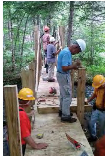
Pete Stapleton (left) and Tom Bryden stand in the stream to screw down deck boards. During this project’s hot weather, they all should have been sitting in the creek!
