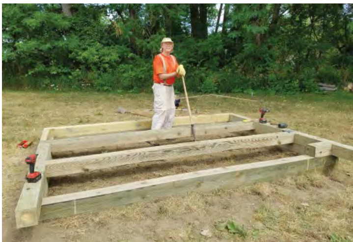
Don Sutherland on top of the base for the shelter that he built of pressure-treated wood.
