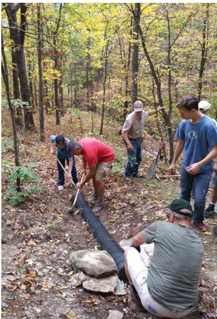
Digging a trench for a drainage pipe to get water off the trail.
