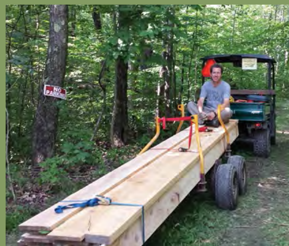
Hemlock posts milled by Mahlon, carried in to the site on our Nova Jack trailer, and pulled by Lynda's Mule.
