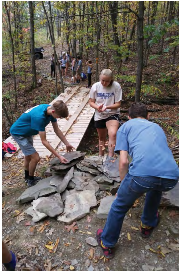
Rock assembly line to "pave" the approach to the bridge.
