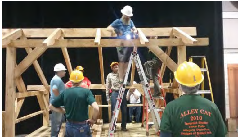
These are the framing beams for Rob Hughes' delightful design, still missing the front rafters. Each board is sanded smooth, with peg holes already there, angled cuts done. Like Mike said, it's a work of art.
