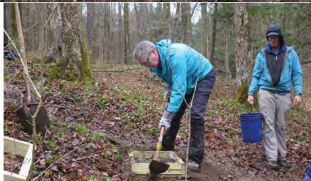
Constructing a box step at the turn of a switchback leg.
