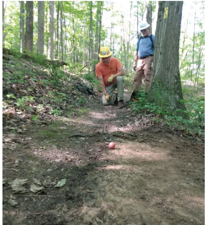
Ed Benson rolling ball to gauge outslope, to ensure that this trail will shed water instead of keeping it on the trail. Good idea, and so simple.
