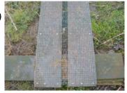
keep puncheon "floating" on the surface. Hardware cloth is bent around sides of stringers and fastened with staples or nails. Although called a 'cloth,' the material is actually metal – threads of hot-dipped galvanized steel "woven" into a mat of small squares (½" size squares recommended).
